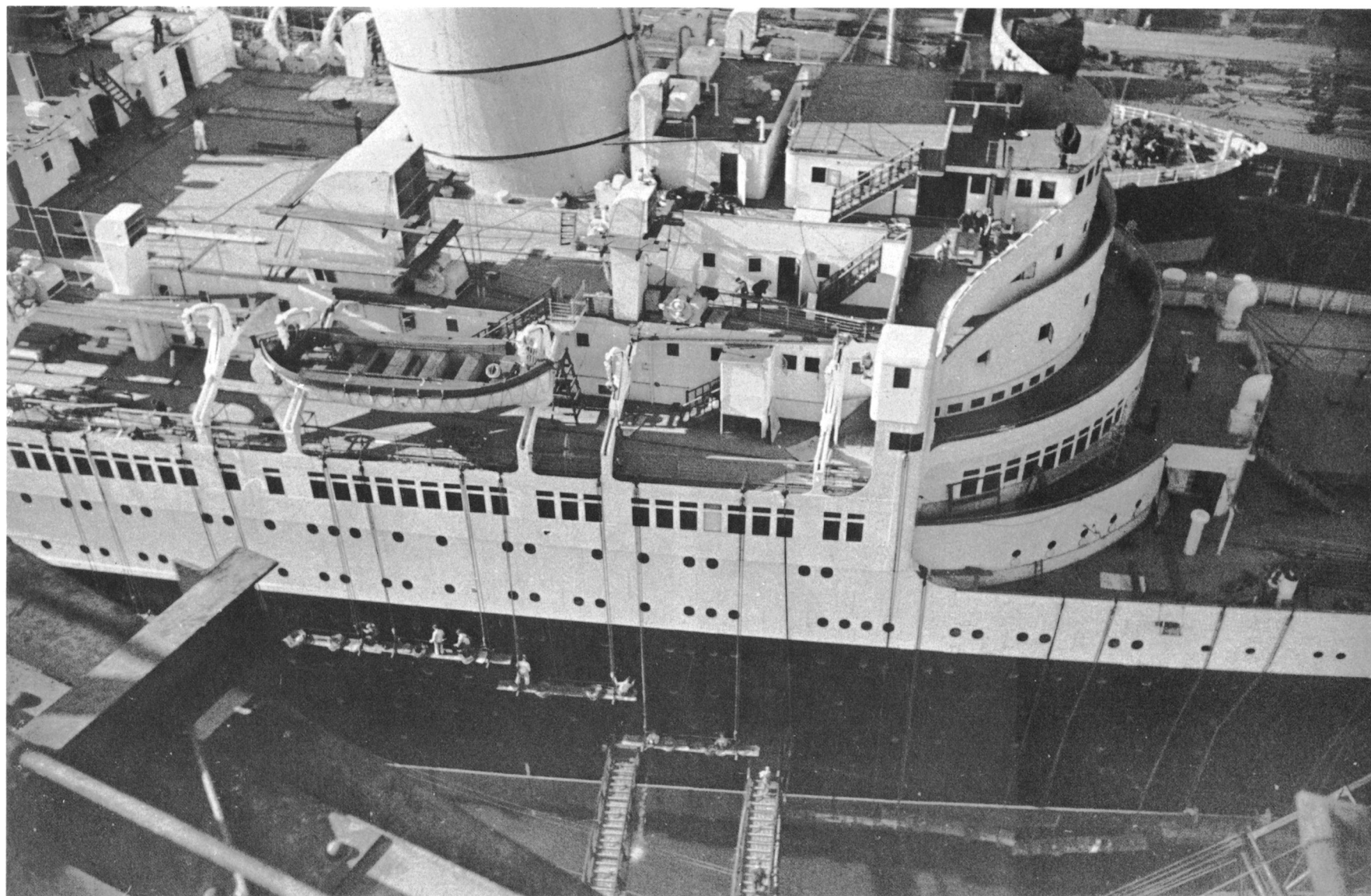
3. View of the forward superstructure during fitting out. Doors for access to the space under the false flooring are especially visible around the forward superstructure just above the sundeck. Popperfoto
