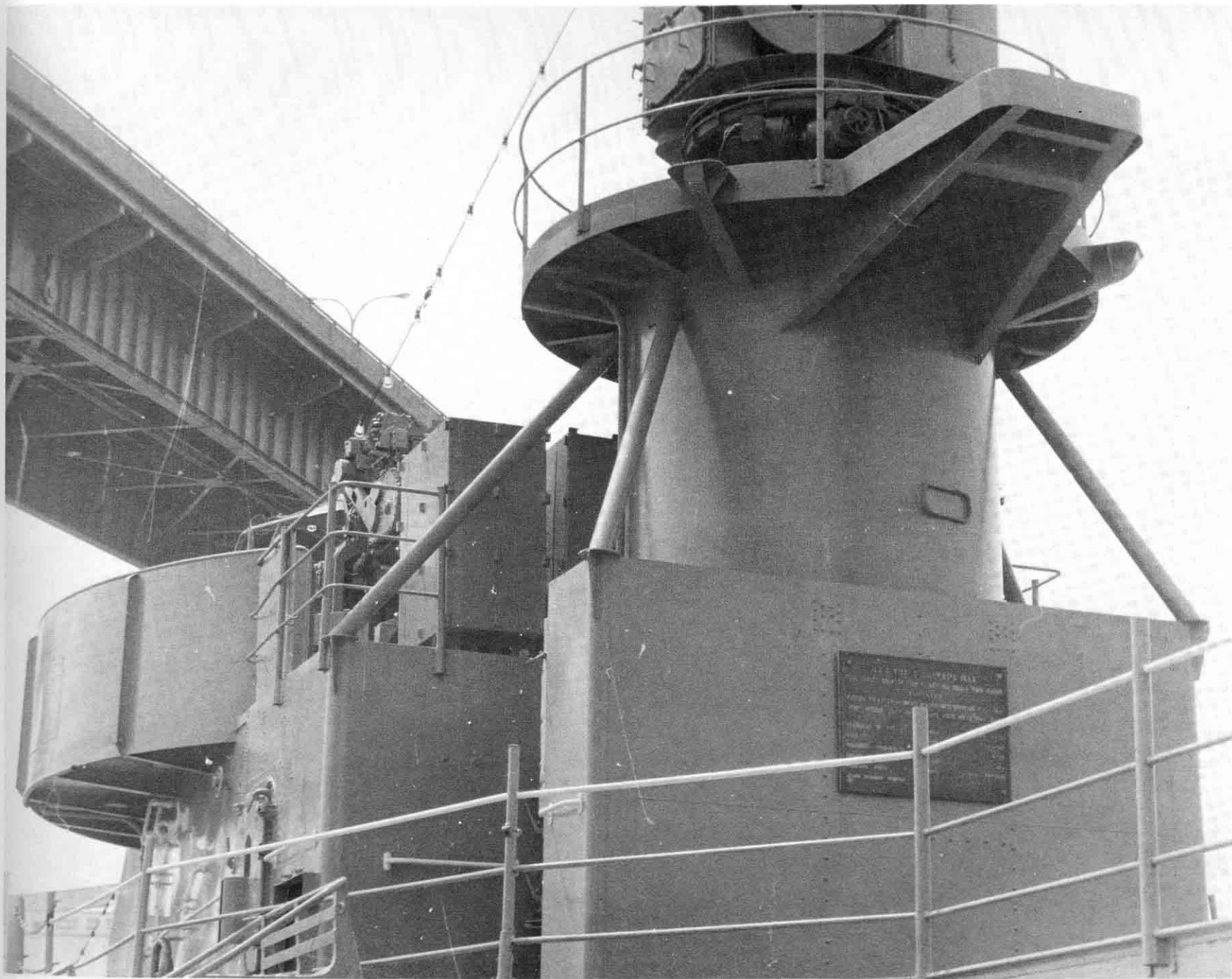
9, 10. These two shots show off the aft 3in/50 platform and its associated Mk 56 director and tower. The rectangular frames along the deck edge held inflatable liferafts, which superseded the floater nets of World War II. The heavy tubular frame just below the gunshield is the aft refueling-at-sea station, the standpipe for
