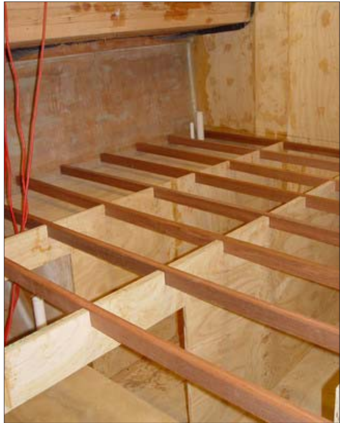
Here we see the sole framing in the raised area in the pilot house. There will be considerable useful room under this sole area so do not forget to allow for adequate access via hatches.
