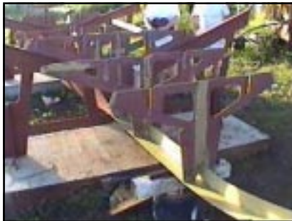
Floor webs being tacked to keel. Note the lightening holes and the notches for sole supports and stringers.
