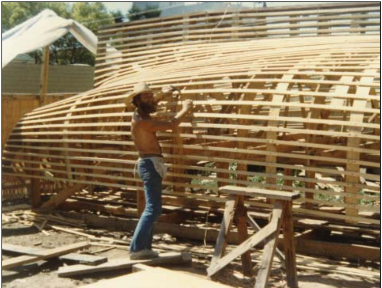
This batten mould for a fiberglass Spray 33 was built in California and illustrates how complex shapes such as the hollow heel at the transition of hull and keel are easily handled using this male mould method.
