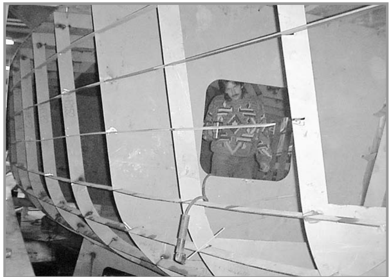
Note the fair line of the stringers as they are installed into pre-cut slots.
