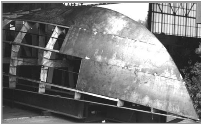
On smaller frameless designs like this one, it may be simpler for the less-experienced steelworker to build a frame from timber.
