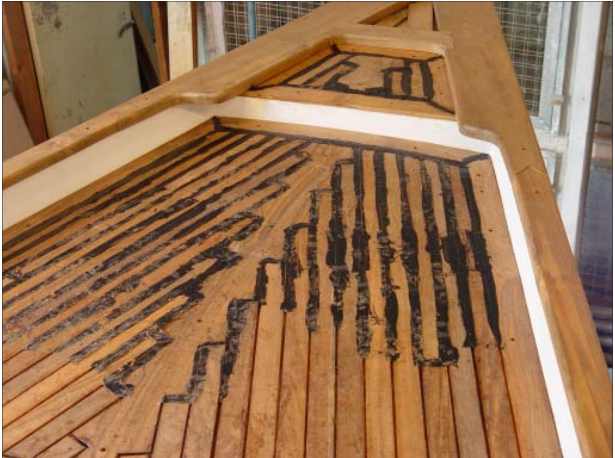
This section has the caulking material applied - Later all will be sanded to give the desired finish.
