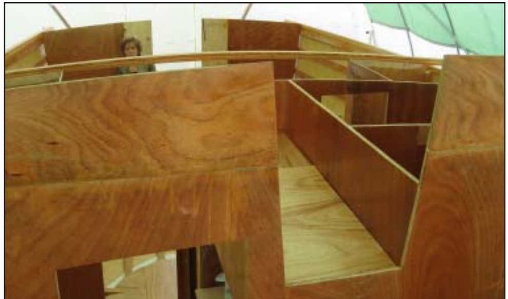
We are looking forward to where the pilot house will be installed - note the pilot house raised sole.
