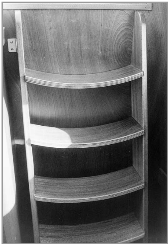
These light companionway steps are practical and reasonably easy to construct.
