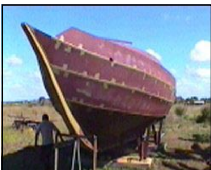
Frames and bulkheads starting to be erected.
