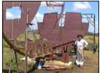
Bulkheads erected and braced. Each kit has a minimum of three steel bulkheads supplied as part of the package.
