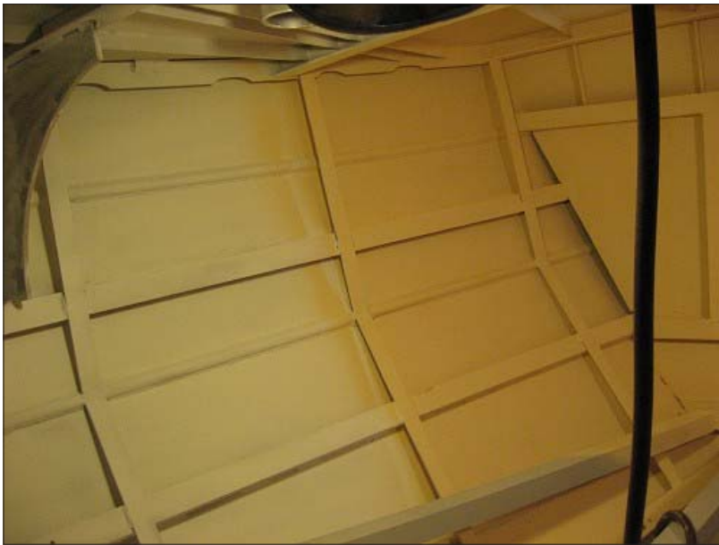
LEFT: Another view of some of the interior coating.
