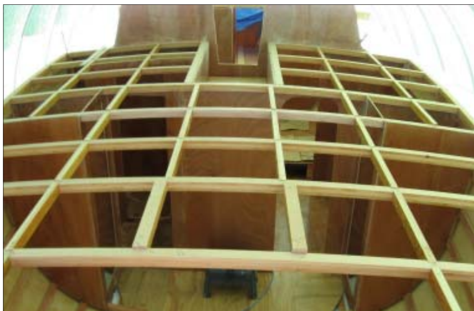
Here we see the laminated deck beams in the flush deck area; note the fore and aft intercostals that are added between the beams. This area will gain much of its strength from the laminated layers of plywood that are used to form the deck structure.
