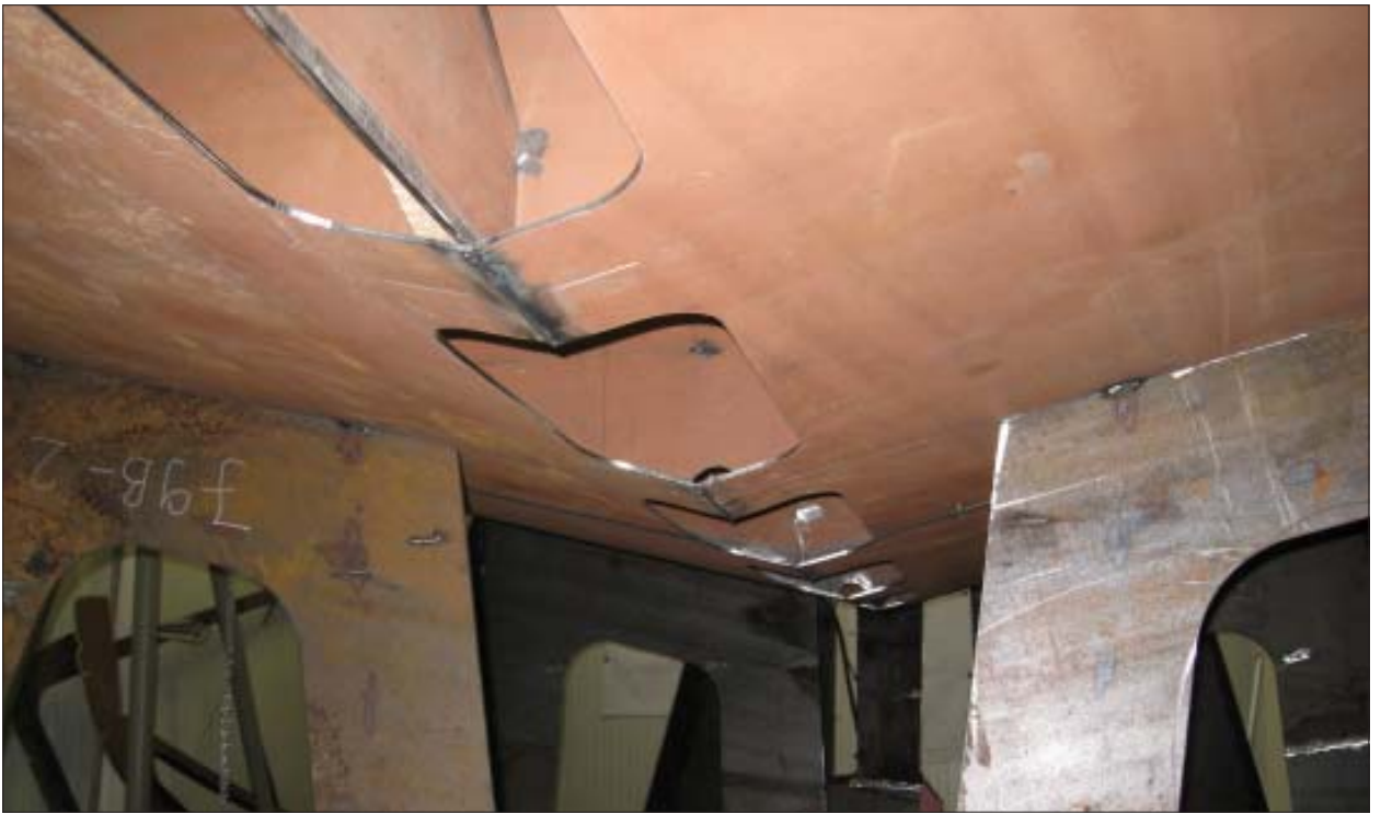
ABOVE: Here we see one frame with a web floor, cabin sole bearer, bottom plate and stringers as well as part of the centerline web. Note the flat bar attached to the inside of the frame.
