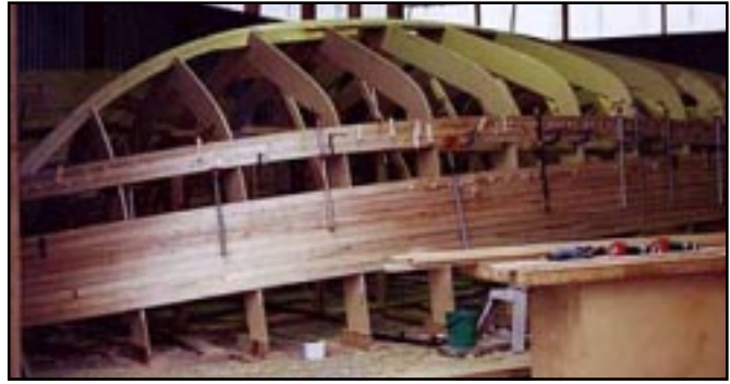
'Stealer' planks are often required to keep the planking on an even keel.
