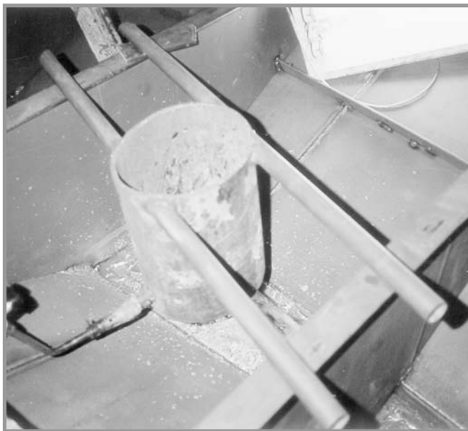
This homemade lead-melting device is fine for installing the final, relatively small amounts of molten lead used to bind the lead pigs into one mass.
