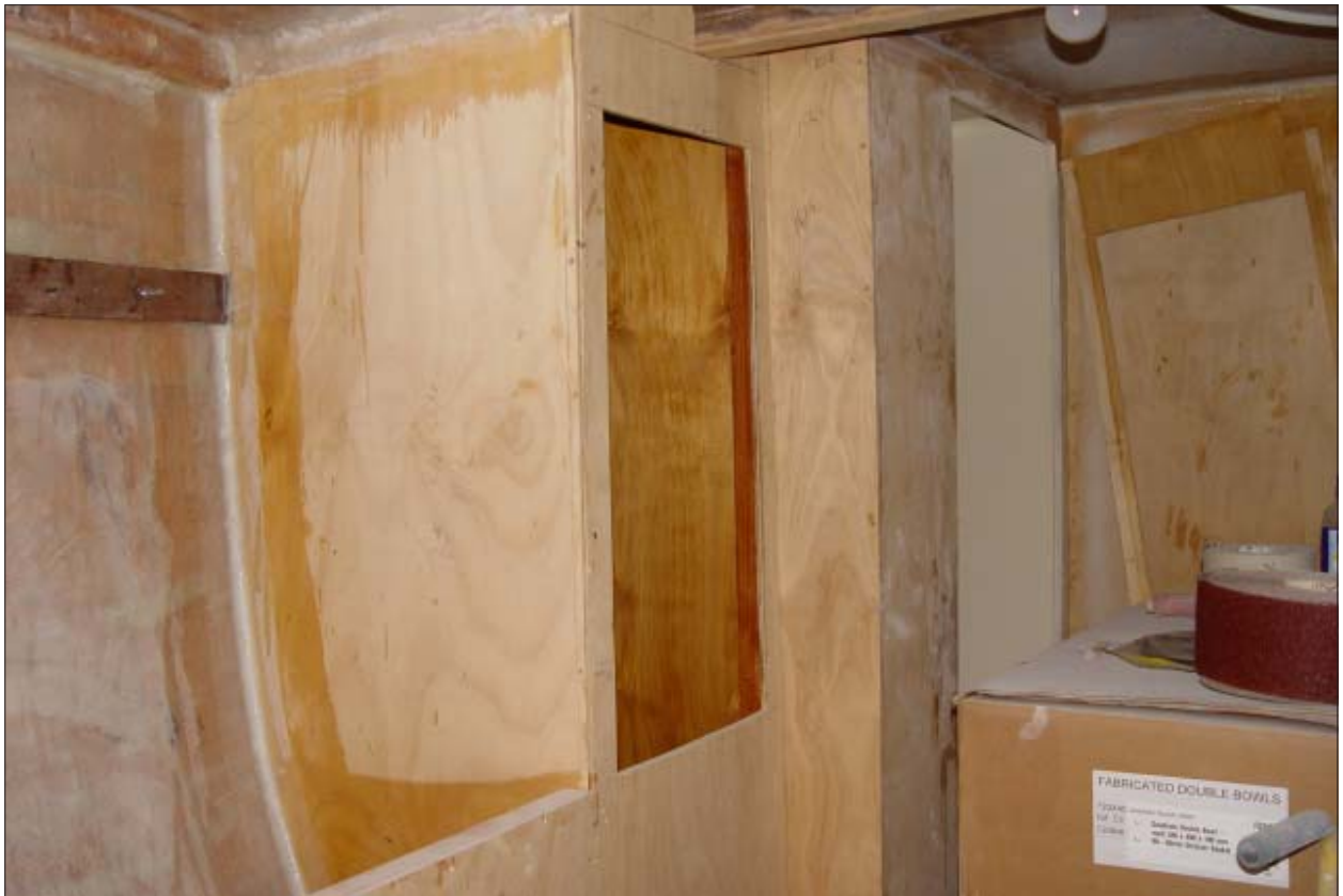
Here we see some of the interior joinery. Note the neat bulkhead attachment to the hull; if properly thought out and carefully installed the lockers, berths and other interior joinery can add an enormous strength to the hull of any boat.
