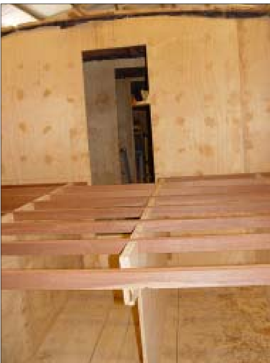
Another view of the pilot house sole area with the forward cabin bulkhead in place; the framing of the pilot house windscreen is just visible at the top of this photo.
