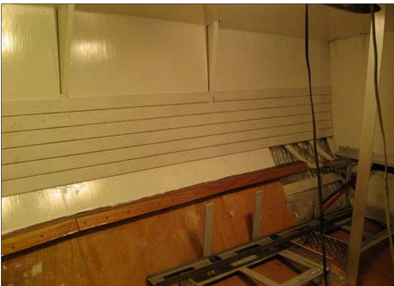
LEFT: The strips are now in place; bet- ter known by the misleading name of ceiling planking!
