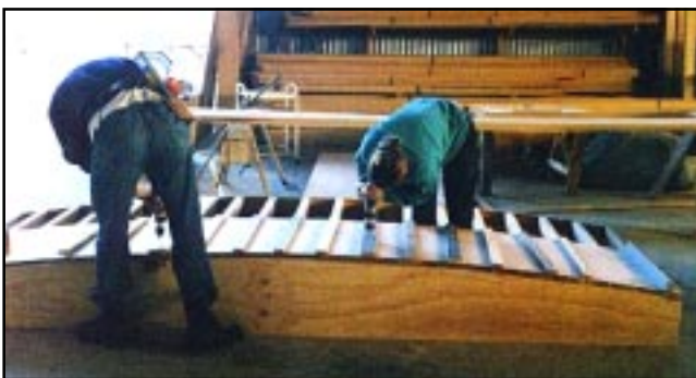
This jig was constructed to laminate various part of the boat. If you plan ahead you can make the jig multi-purpose; here it is being used to laminate part of the transom. Photograph by permission of Rob McGill and Nina Morissette,
