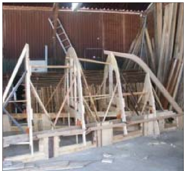
Above we see Graham taking off the frame shapes from the full size patterns and getting started on setting up the hull framework.
