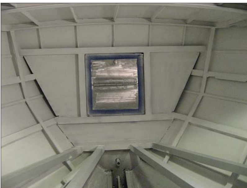
LEFT: Nice even finish; even though it will be covered up with the interior joinery etc., make every step the best you can manage.
