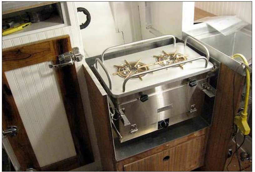
RIGHT: The neat installation of the stove shows a lot of thought has gone into this area.
