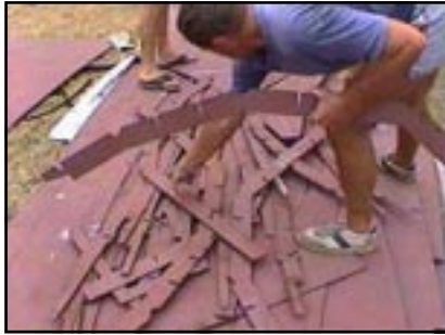
Frame part showing limber holes and the pre-cut slots for the stringers to sit into.
