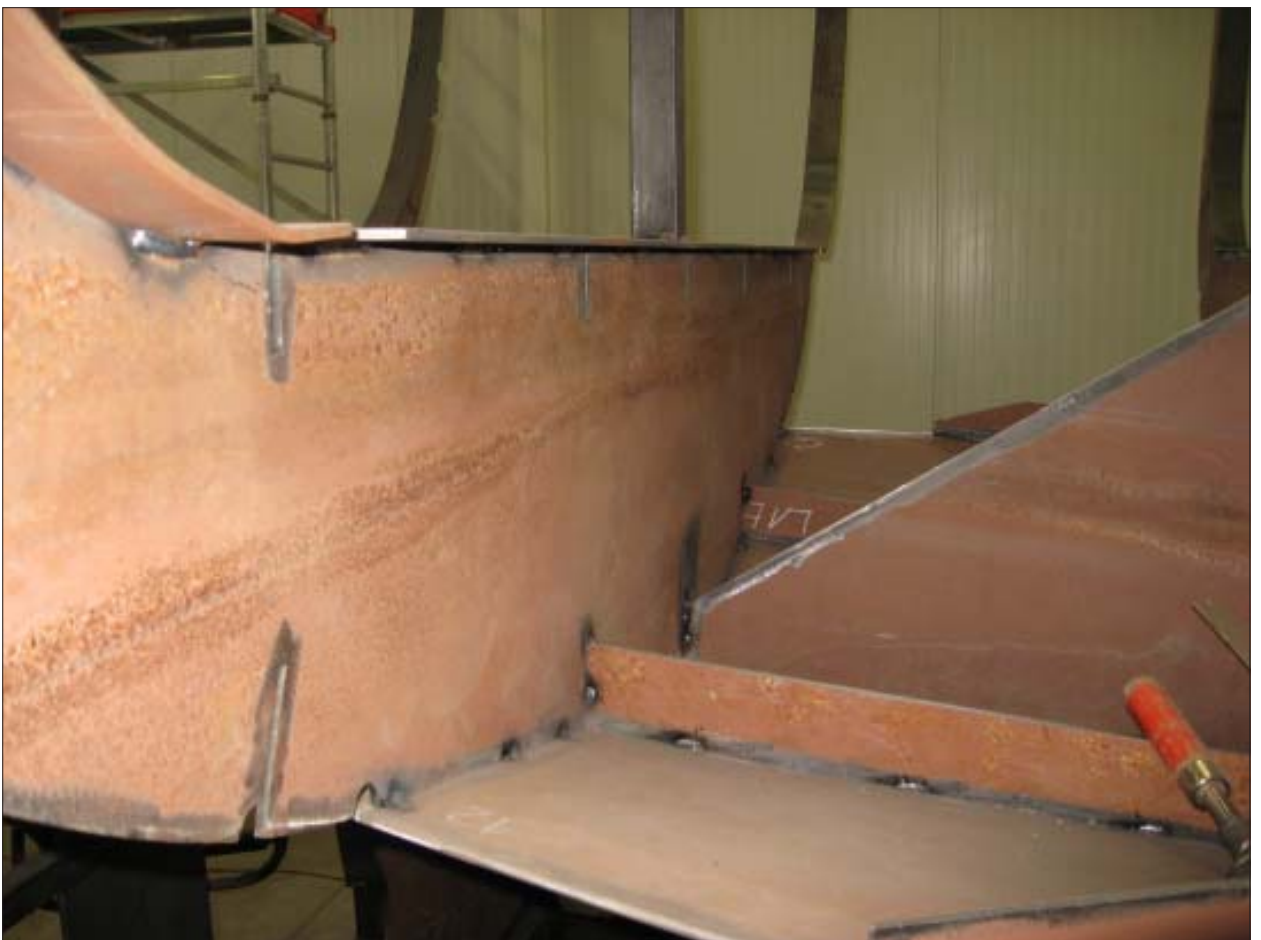
ABOVE: This photograph shows the bottom plates supported in the setting up jig. The hull could be better supported by using a strip of flat-bar across the top of the supporting jigs so as to spread the load between the bottom plates and the jig; this would also strengthen the setting up jig which will take a considerable weight before the hull is completed.
