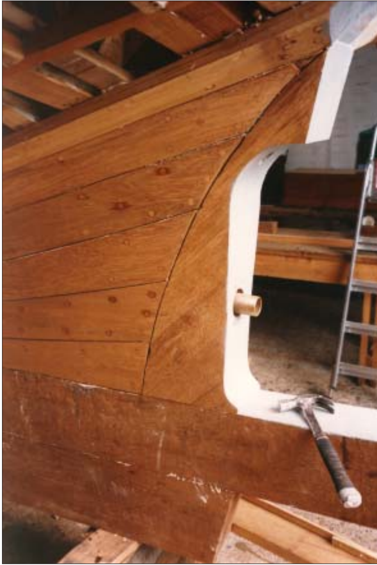
Note the heavy keel timbers, heel, stern tube, steam bent frames and temporary stringers that will be removed as planking proceeds.
