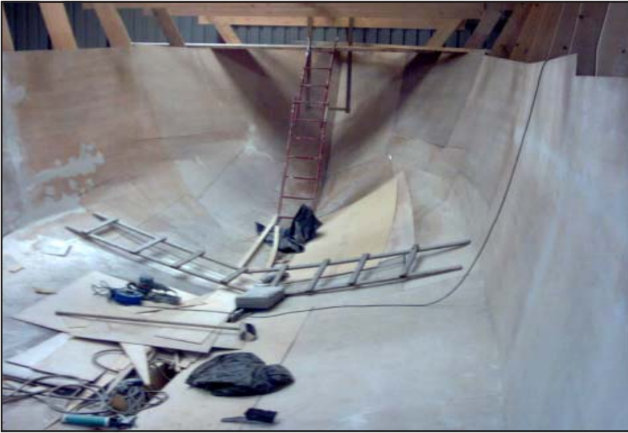
Here we see the mould lining installed in a chine hull mould.
