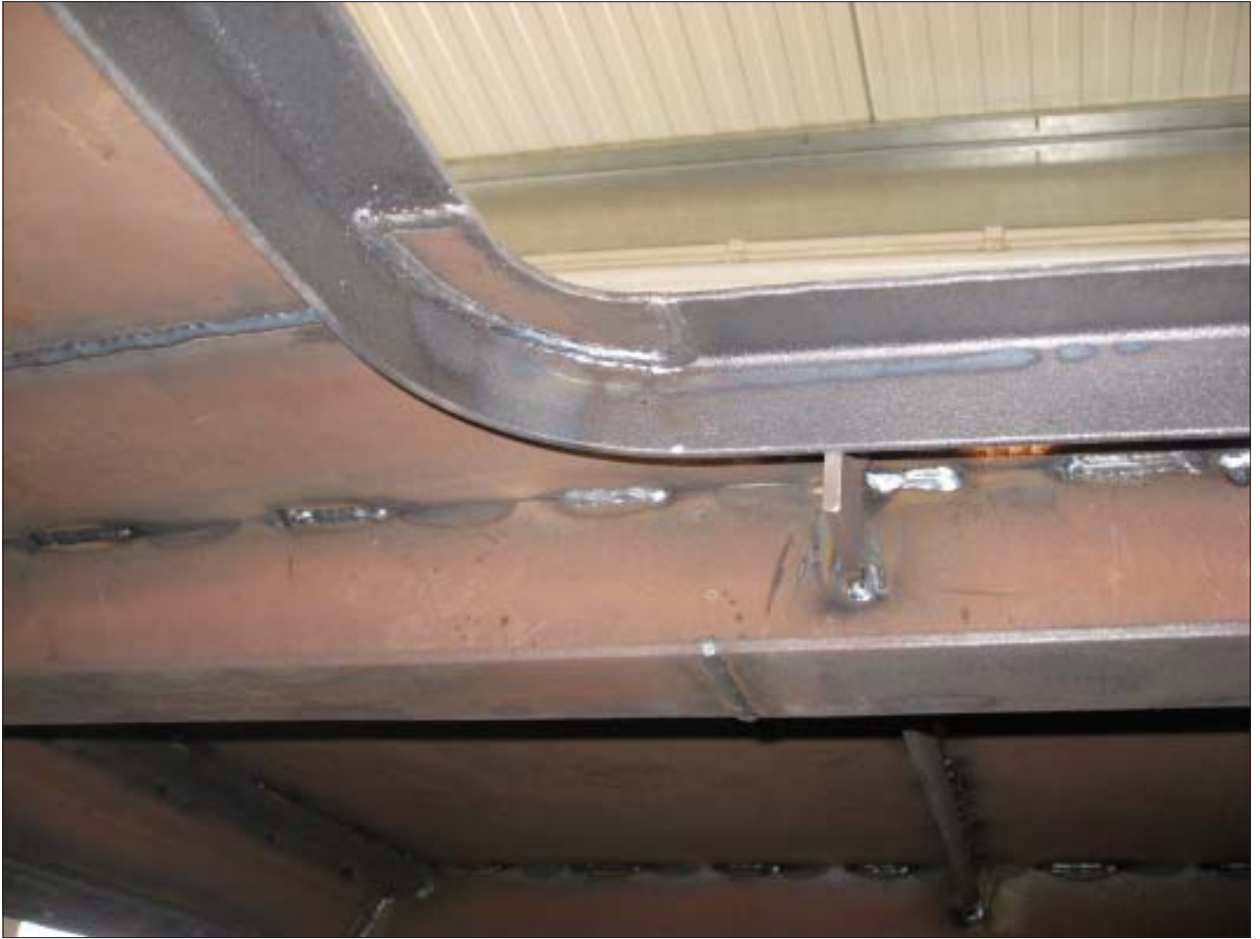
ABOVE & BELOW : Two views of the hatch frames on place.
