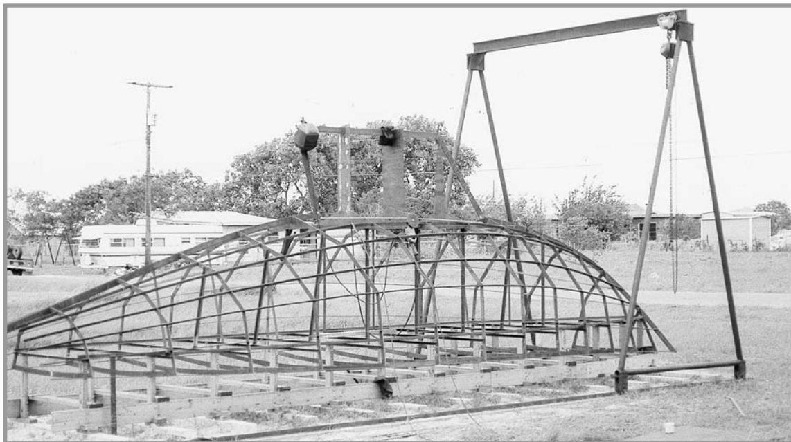
An overhead gantry set on rails can make the handling of plate a much easier and safer operation.
