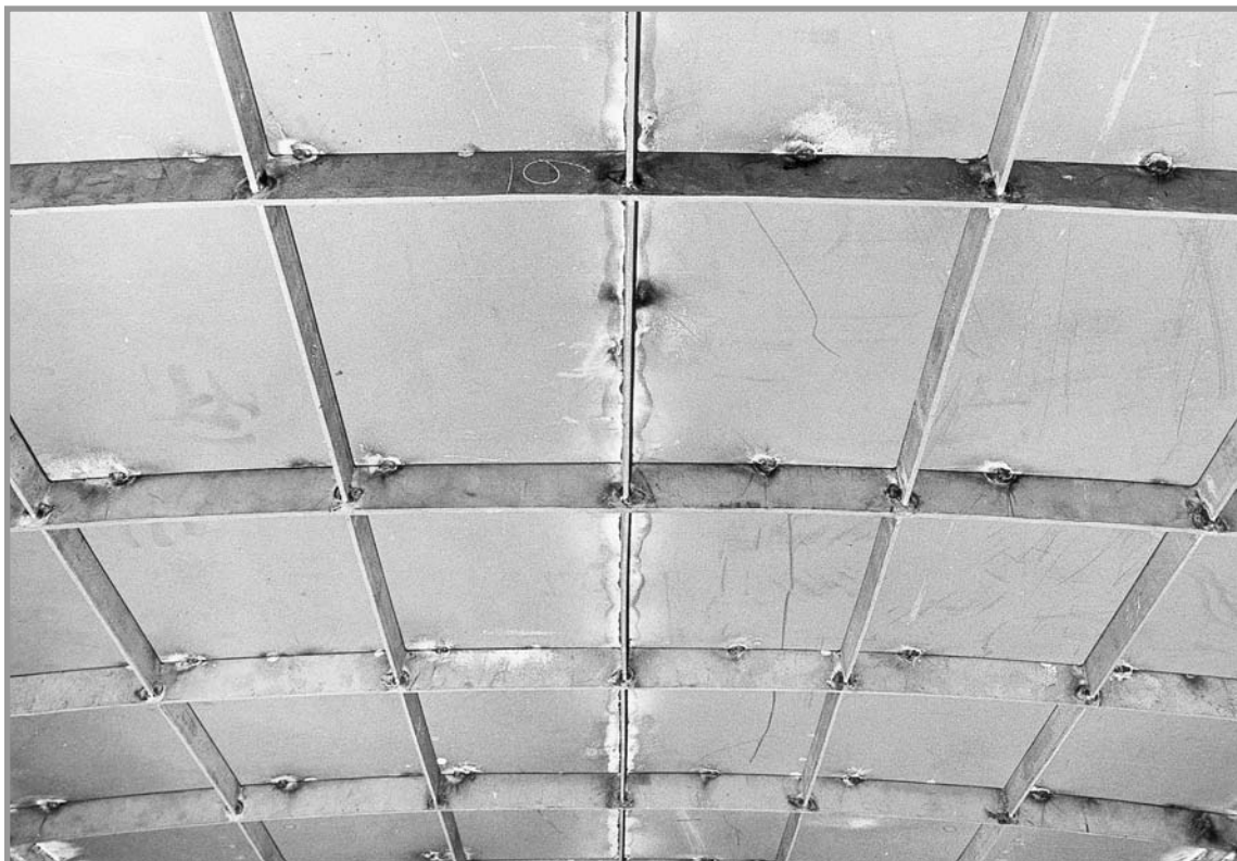
Cabintop beams and fore-and-aft intercostals tack-welded in position; see text.
