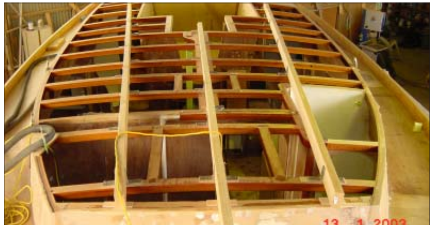
Cabin top beams that were pre-varnished before the cabin top was installed.
