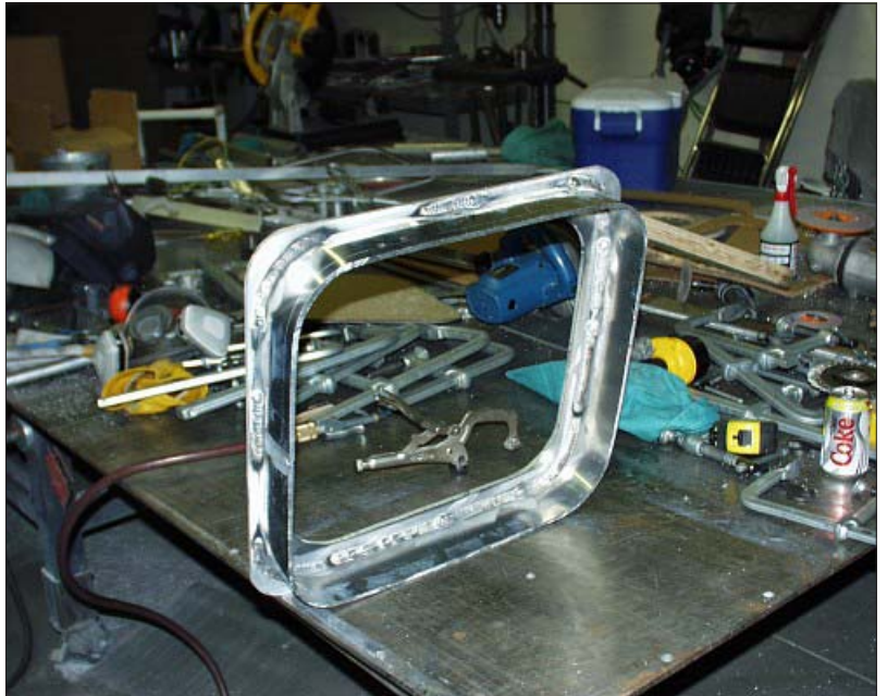
RIGHT: Here the preparation of the window frames for the pilot house sides is going well.
