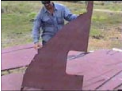
Forward bulkhead. By studying the cut out shapes on the plans beforehand, all parts are readily identifiable.
