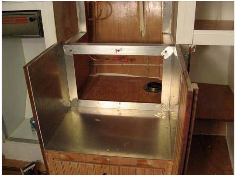
RIGHT: In this case the builder used a mix of aluminum, timber and plywood to achieve what looks like being an attractive fit-out.
