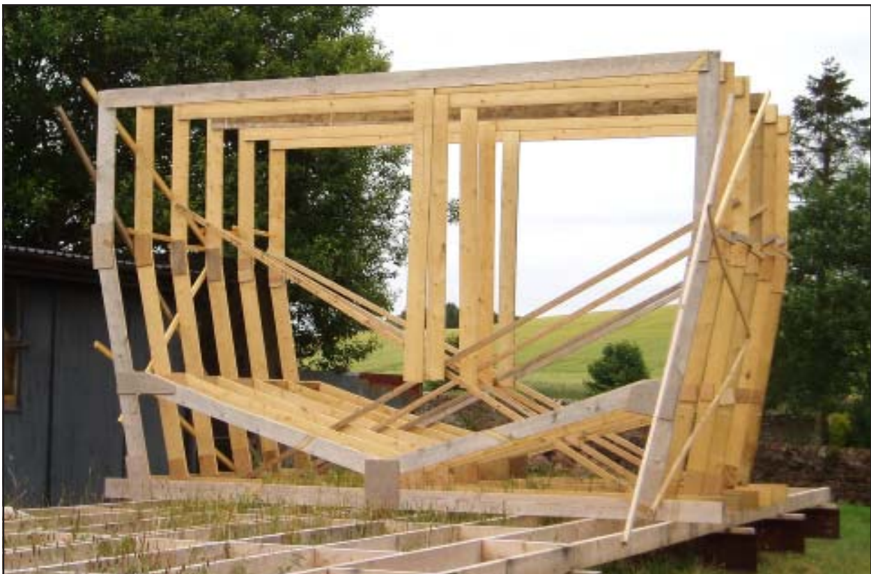
After assembling all the frames, they are set up on a system of bedlogs.
