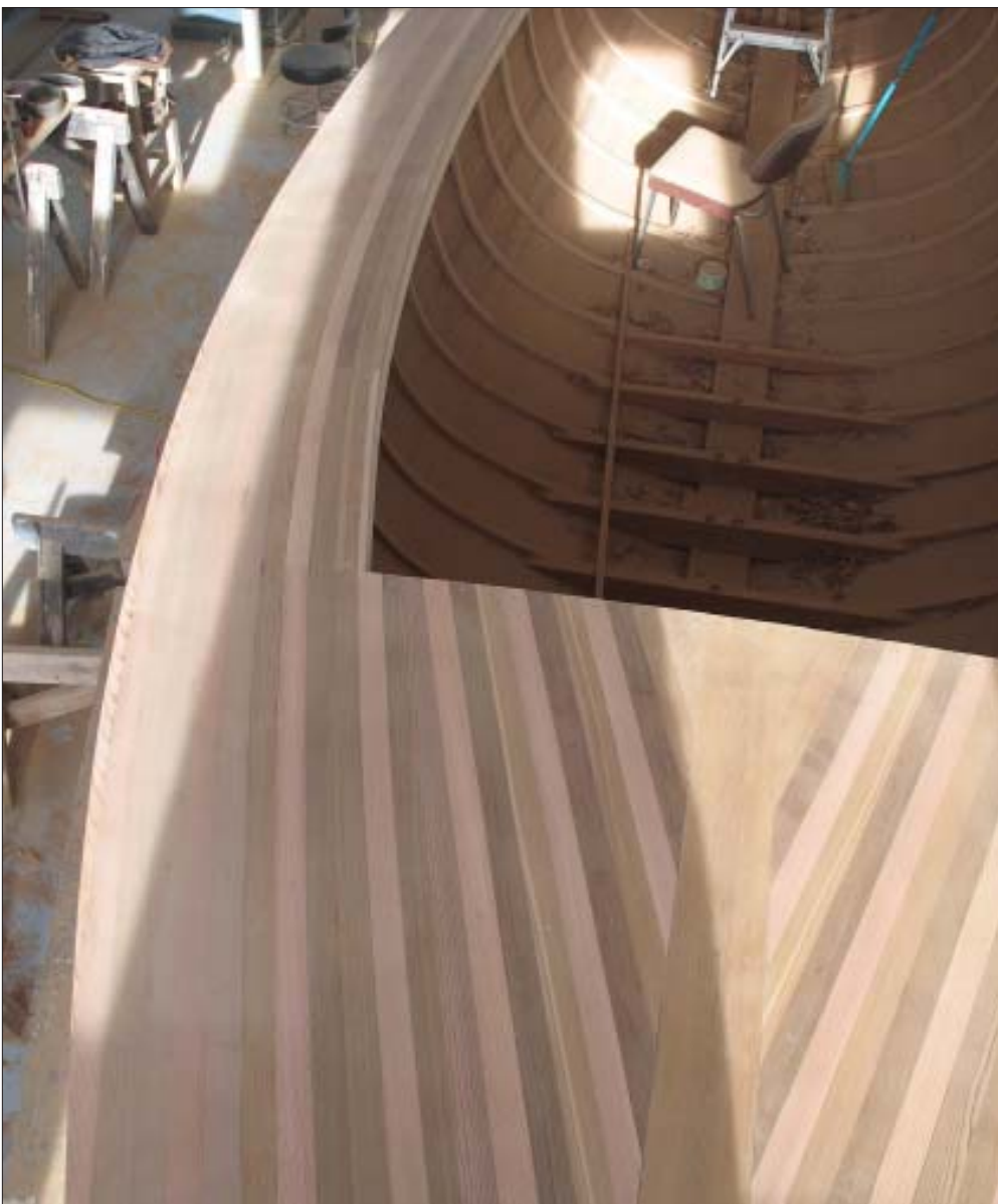
LEFT & ABOVE This is a Wood Epoxy Roberts 246 built using the strip plank technique. As you can see the builder is making a very nice job of building this hull and deck. Note the cast lead that has been bolted to the timber keel.
