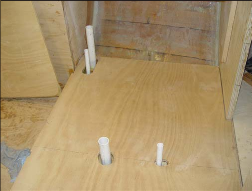
More tanks with top and pipes in place.
