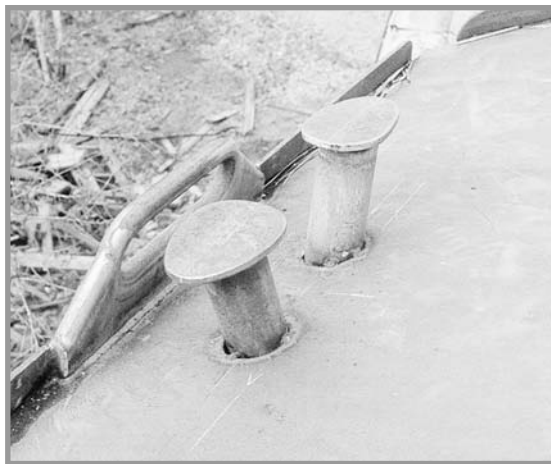
This bollard and fairlead combination works well; it would be improved if built from stainless steel.
