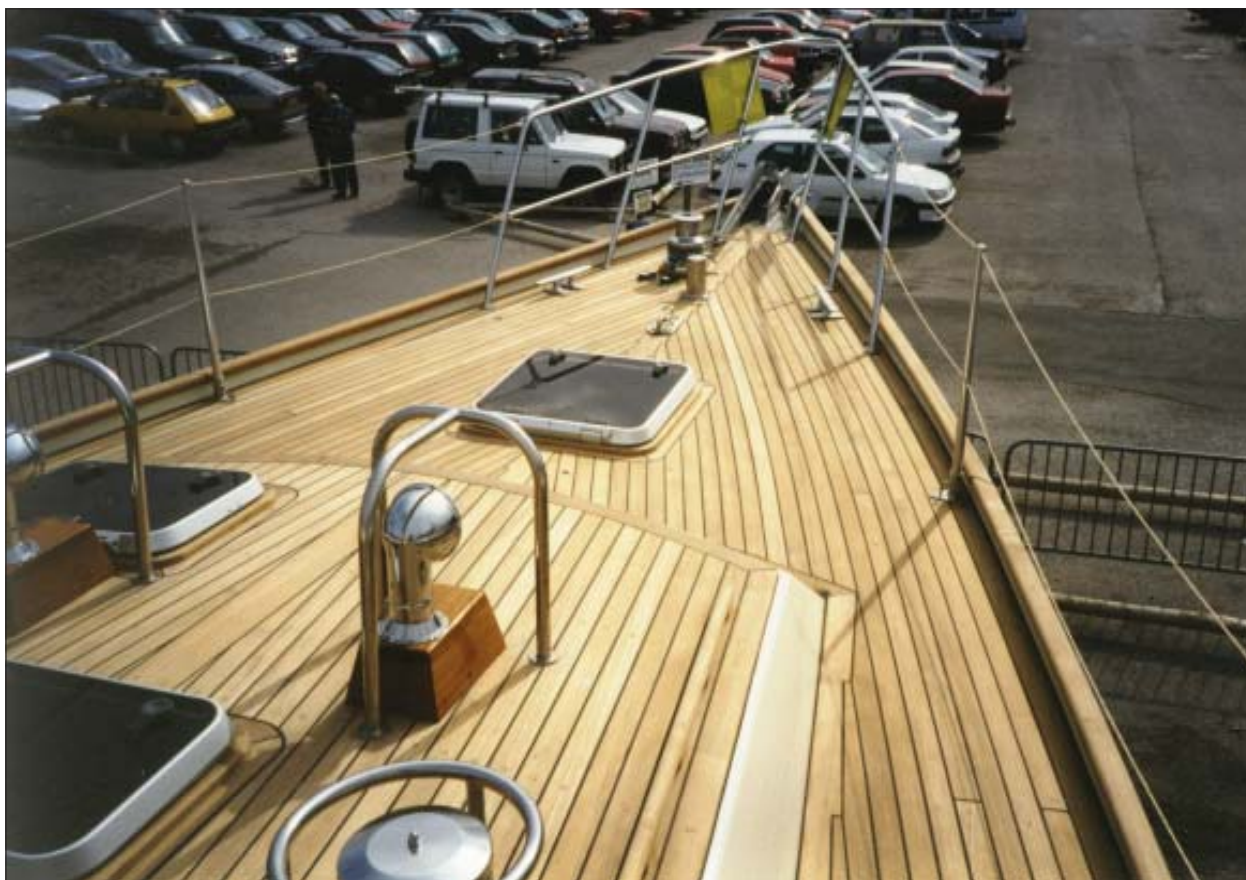
This teak deck is installed on a Roberts 432 built in the UK and is a good example of what can be achieved by careful planning and layout combined with fine workmanship as shown here.
