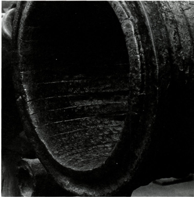
The muzzle of a wrought iron bombard in the collection of the Museu Militar, Lisbon, showing hoop and stave construction. Forged in Goa in 1518, it fired a 200-pound stone ball. The staves were hammer-welded together around a wooden mandrel; the reinforcing hoops were then heated white hot, slid over the staves and hammer-welded into place as they contracted. Corrosion has accentuated the welding joints; they would have been barely visible when new.
