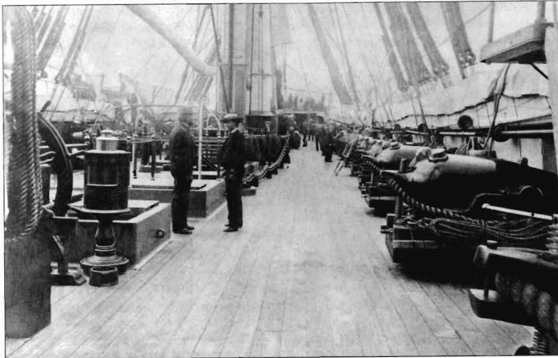
View on gundeck of US Navy screw sloop Hartford , 1864, showing Dahlgren 9-inch shell guns in broadsides. (Naval Historical Foundation, NH 53678)
