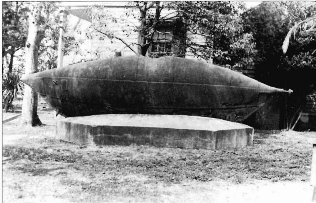
Pioneer , Confederate Navy submarine. The propeller vanes are broken off and the hatch or conning tower is missing. (Louisiana State Museum, New Orleans. Naval Historical Foundation, NH 42854)
